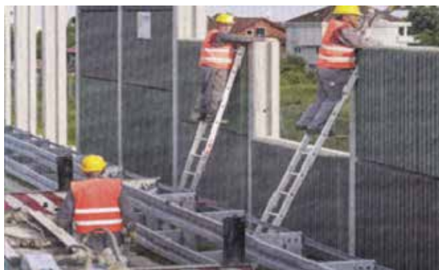
Figure 23. Noise barrier type Ruconbar (Croatia)
