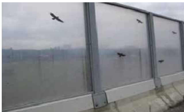
Figure 20. Noise barrier at Skopje bypass
