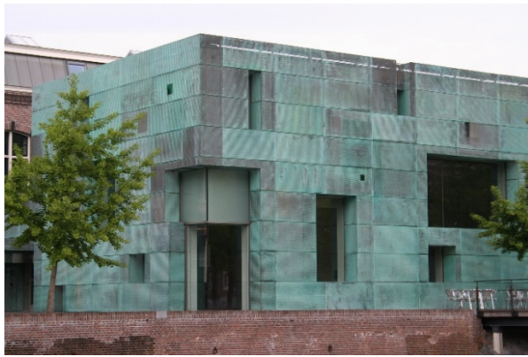
Figure 3: Detail of Facade, Sarphatistraat office – Amsterdam (1999), Steven Holl
