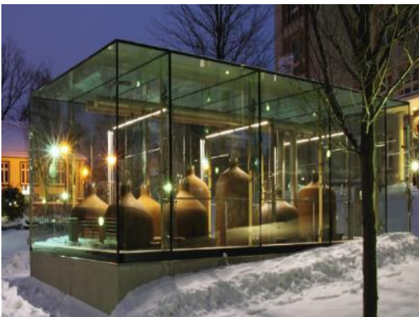
Fig. 7. All glass enclosure at Leibniz Institute in Dresden, Germany [3]
