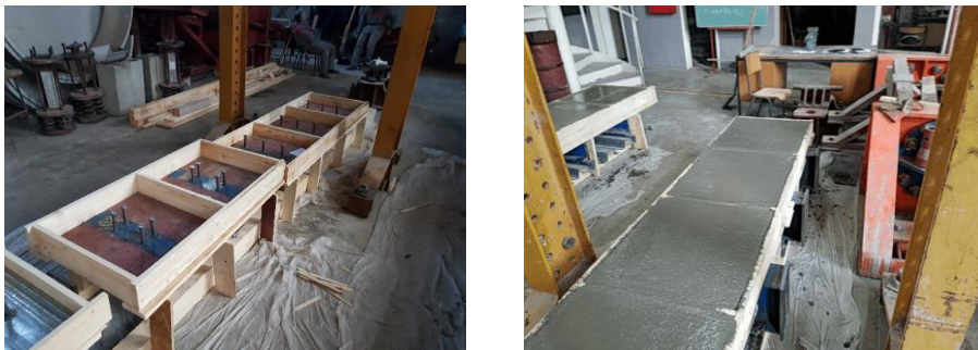
Figure 3. Casting of concrete
