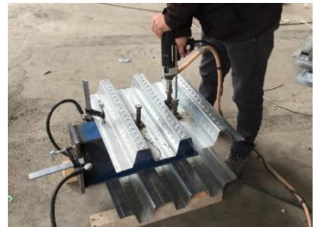
Figure 2. Welding of headed stud
