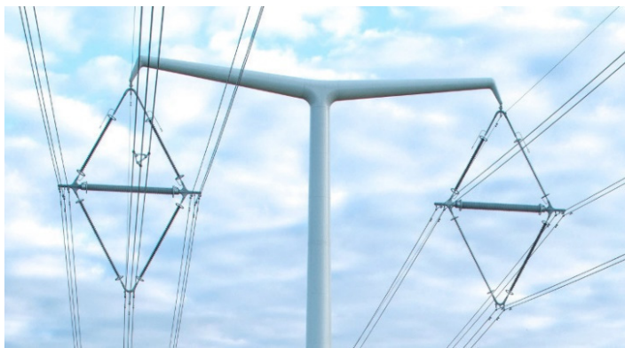
Fig. 2. Steel tubular tower
