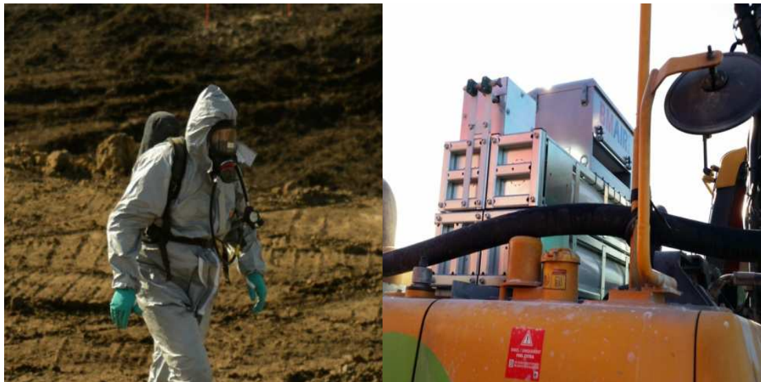
Fig. 5. Left, full set of PPE with self-contained breathing apparatus. Right, compressed air bottles connected to the cabin of an excavator.
