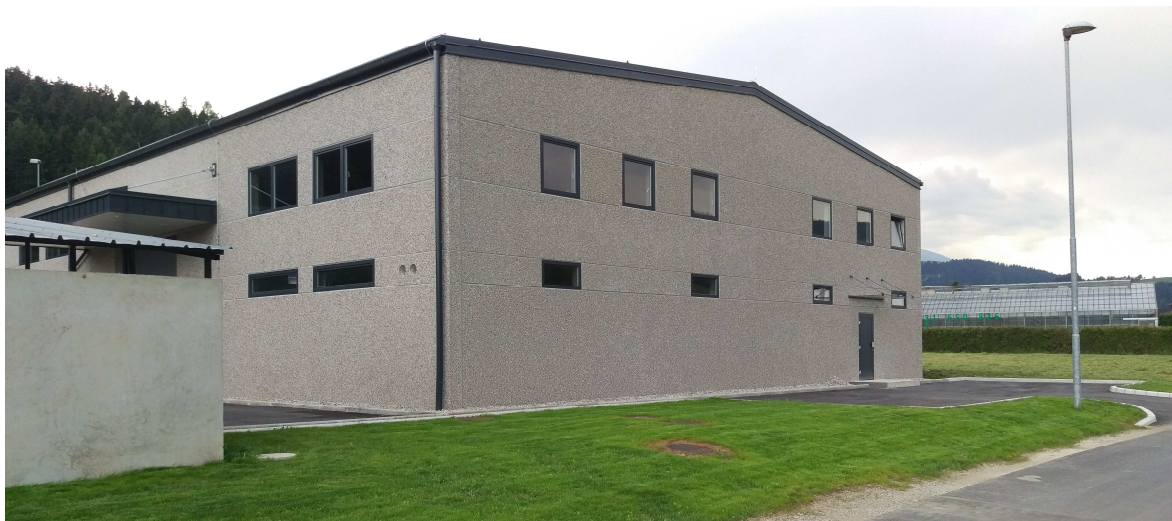
Fig. 2. Demonstration plant for soil washing technology.
