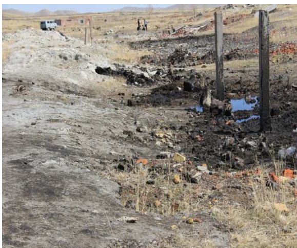
Fig. 3. The ruin of old heating plant in Bayantumen soum
