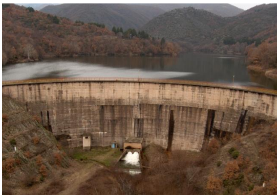
Figure 5. Dam Gradce - Kocani, structure on which is performing auscultation more than 40 years from members of geodetic department
