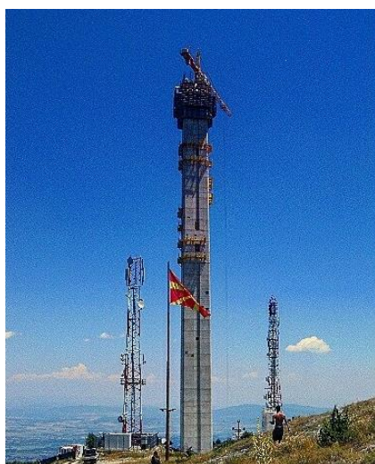
Figure 1. Kula Vodno (in construction)
