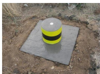
Figure 10. Stabilization of the nodal points
