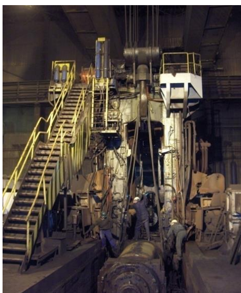
Figure 1: Mill stand construction in hot rolling mill - “Makstil” SC - Skopje
