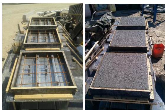
Figure 3. Casting of the concrete
