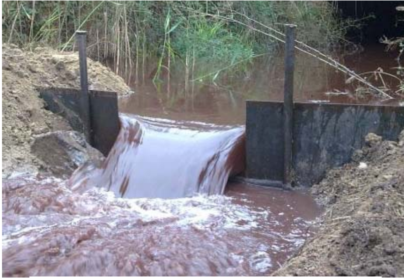
Figure 3. Overflow of MM-0, condition of 16 October, 2009
