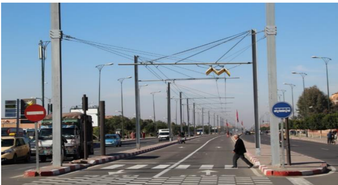
Fig. 9. The eastern end of the catenary section of Marrakesh's BRT system
