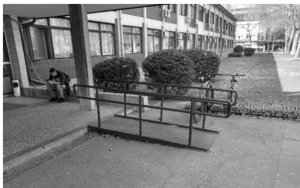
Fig.12. Ramp at the entrance to the Mechanical Engineering Institute building
