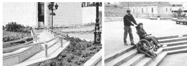
Fig.8. Ramp of big length at the Serbian National Theater in Novi Sad and the usage of a stair climber
