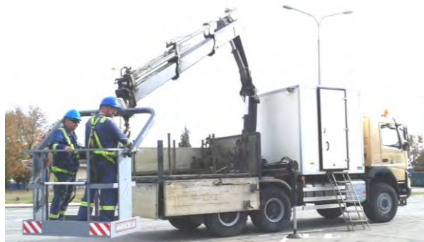
Fig. 1 Elevating persons, IWP attached to a loader crane
