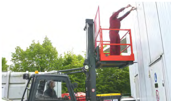
Fig. 2 Elevating a person by means of a NIWP on a CFT, [2]
