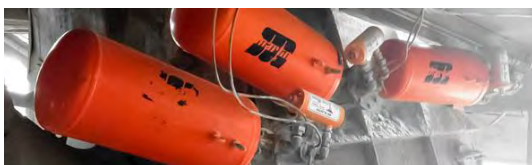
Fig. 10 Air cannons installed on the feeding hopper by the Martin Engineering Company UK
