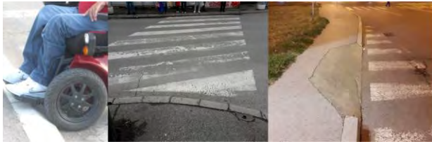
Fig. 2 High curbs in Nis as obstacles for the movement of wheelchair users
