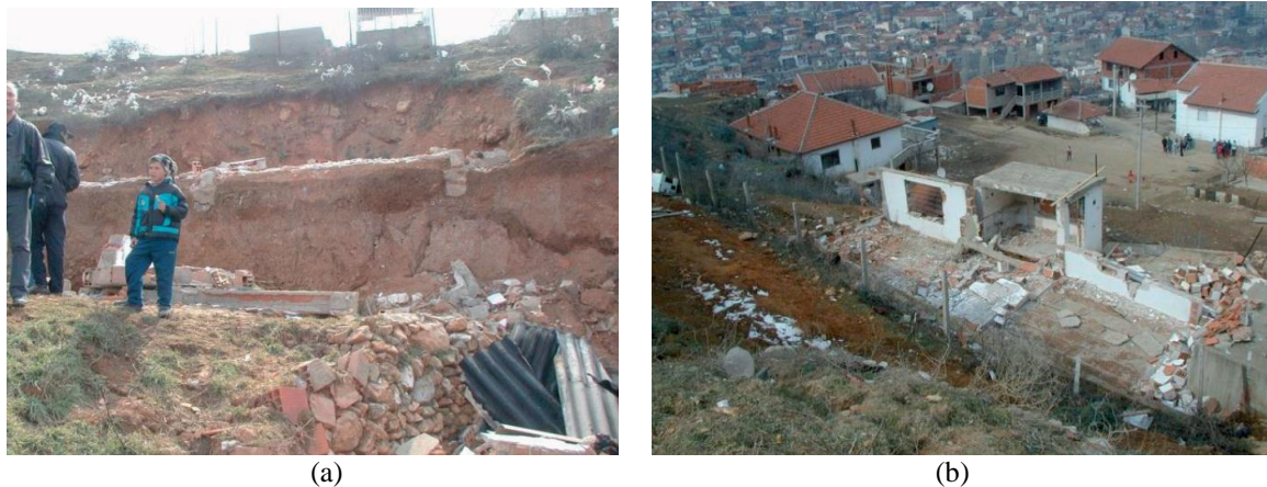
Figure 11. Photo of the (a) top zone of main scarp and (b) buttress zone of the landslide
