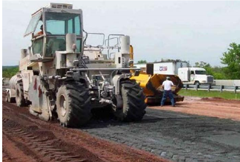
Fig. 2 Mixing of soil and fly ash with recultivator
