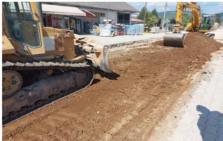
Fig. 1 Excavation of the existing subbase at km 11+000, karpalak - želino section
