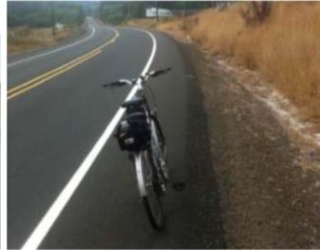
Fig.7. Example of narrow hard shoulder
