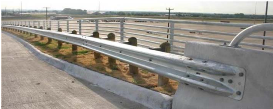
Fig.15. Example of transition between concrete barrier and guardrail
