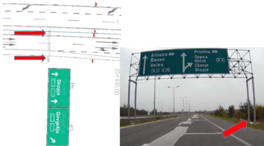
Fig.12. Unprotected portal posts left and right side on chainage
