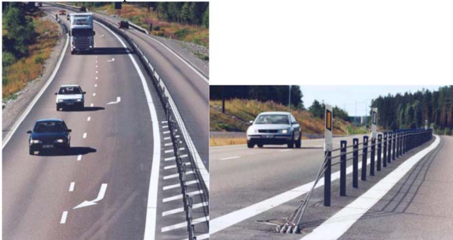
Fig.4. Typical 2+1 roadway with centre cable barrier in Sweden
