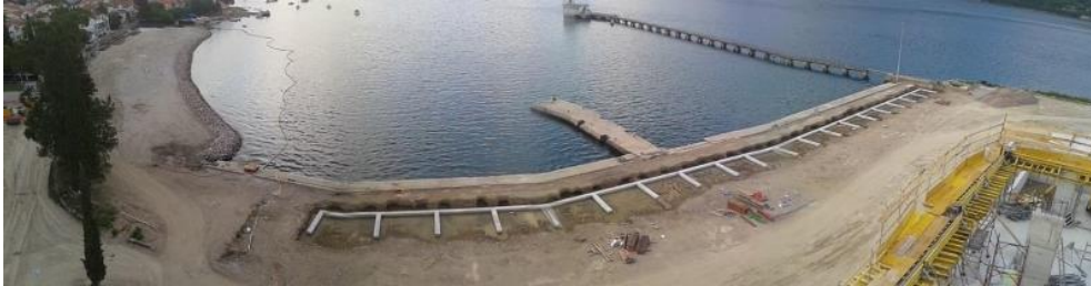
Figure 9. Capping beam of the future West Quay Wall
