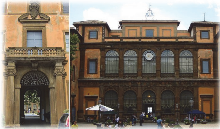
Fig. 58. (left) Entrance to the courtyard; (right) portico and loggia
