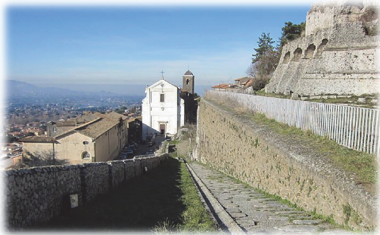
Fig. 71. One of the two ramps leading to Terrazza degli Emicicli
