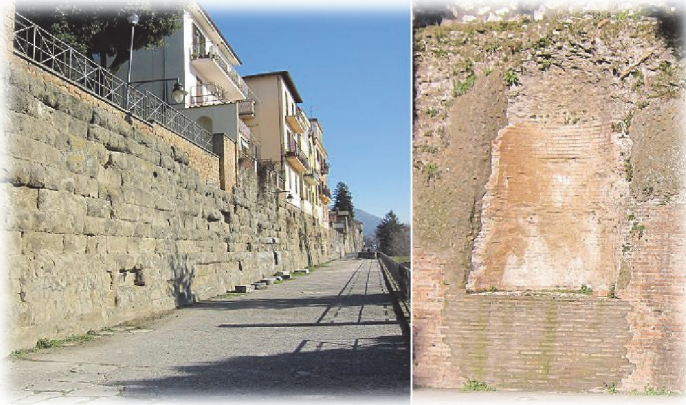
Fig. 66. (left) Walls supporting the third terrace in "opus quadratum"; (right) a brick wall in "opus latericium" forming a niche which was added to the structure supporting the first terrace
