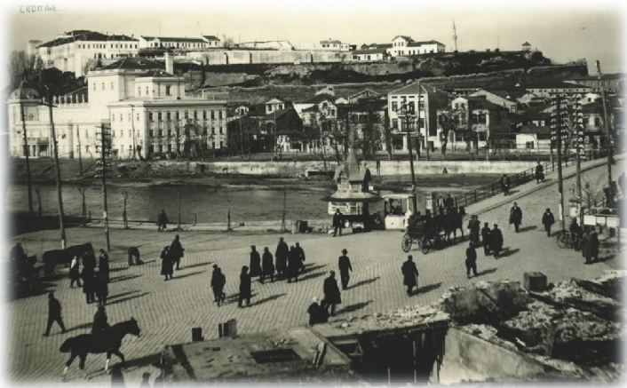
Fig. 16. Skopje 1953: A view of Stone Bridge and Skopje (Kale) Fortress
