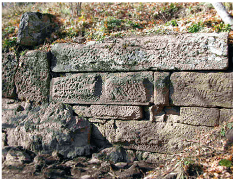
9. Masonry of the walls at Visoka
