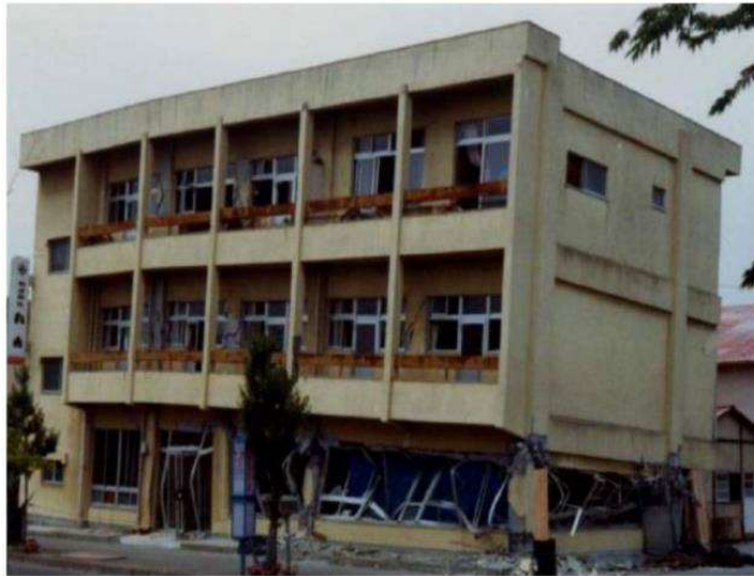
Figure 30 - Damage of three storey building during 1978 Mijagi-Ken-Oki earthquake, [14]
