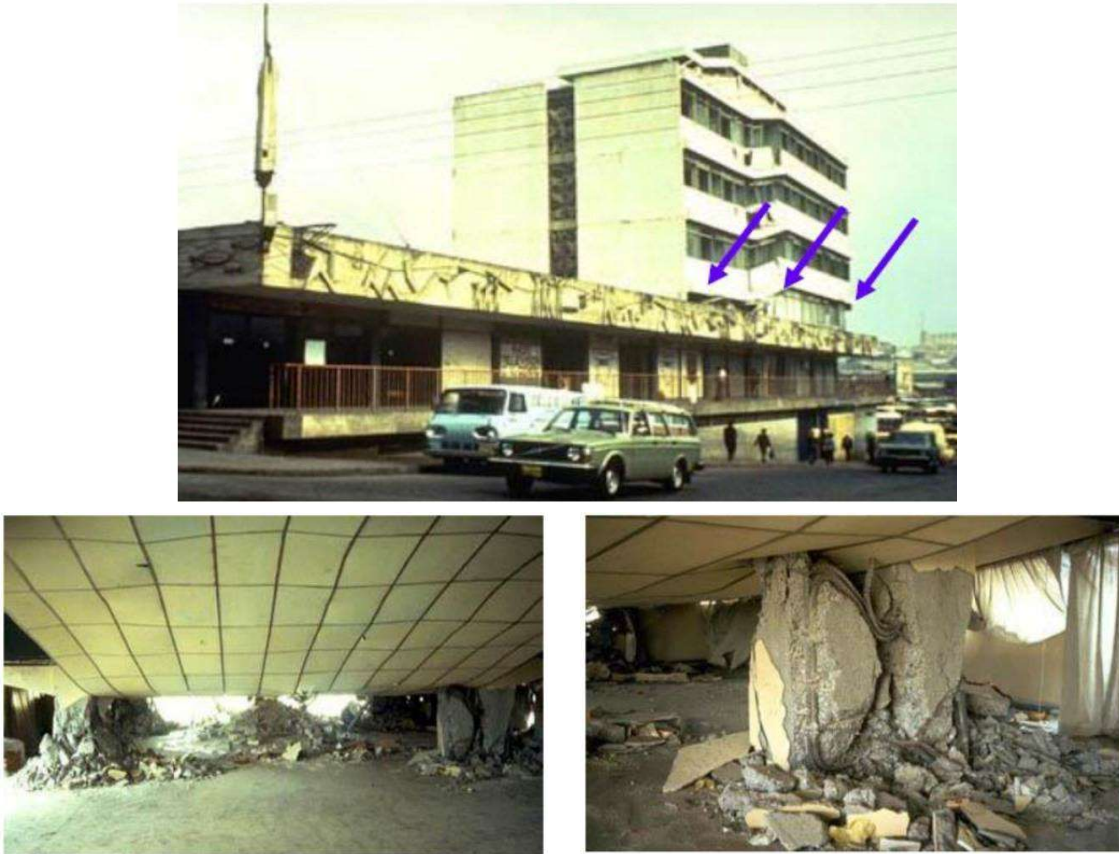
Figure 33 - Damage due to irregularity during Guatemala earthquake 1976, [14]
