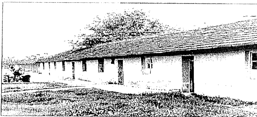
Picture 1. The old building where the Institution began with work
