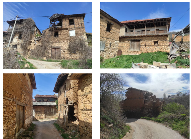
Figure 4: Photos of traditional architecture in the village of Gornjane (characteristic examples)
