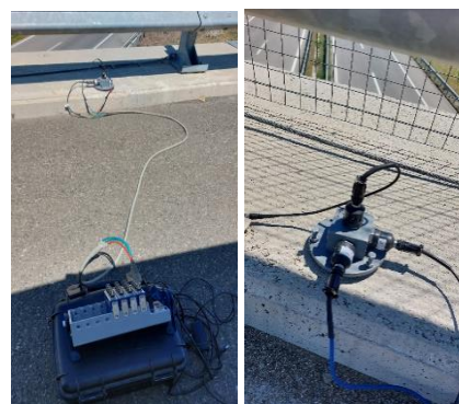
Figure 1. Field monitoring equipment (left), three-way accelerometer (right)
