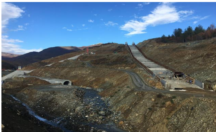
Figure 13. Diversion tunnel exit
