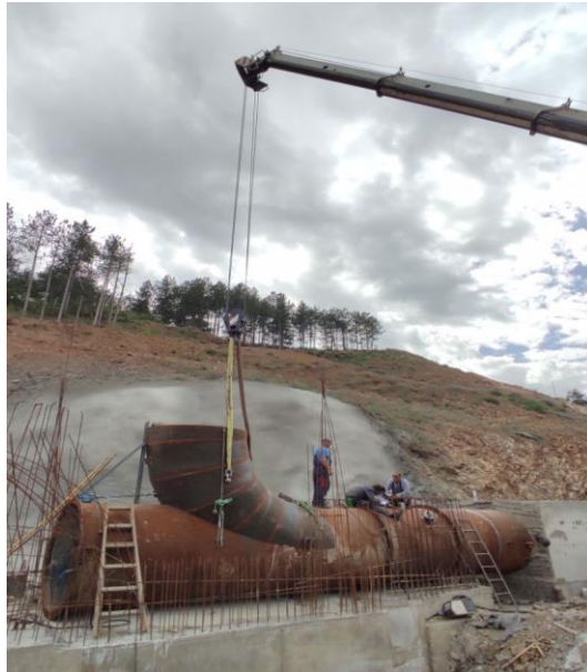
Figure 5. Elbow installation for the connection of entrance construction and steel pipe
