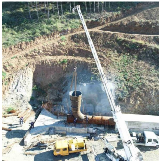
Figure 6. Installation of a cone for entrance construction
