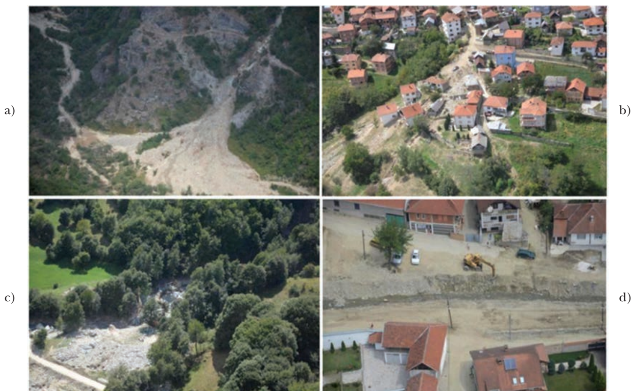
Fig. 4 – Some photo of landslides and impacted infra(structures) during the last catastrophic event occurred on 3 rd August 2015: a) debris fan near small electricity power plant; b) debris flow path through the Shipkovica village; c) debris flow material completely covering the road between Shipkovica and Brodec; d) affected area in Golema Recica.
