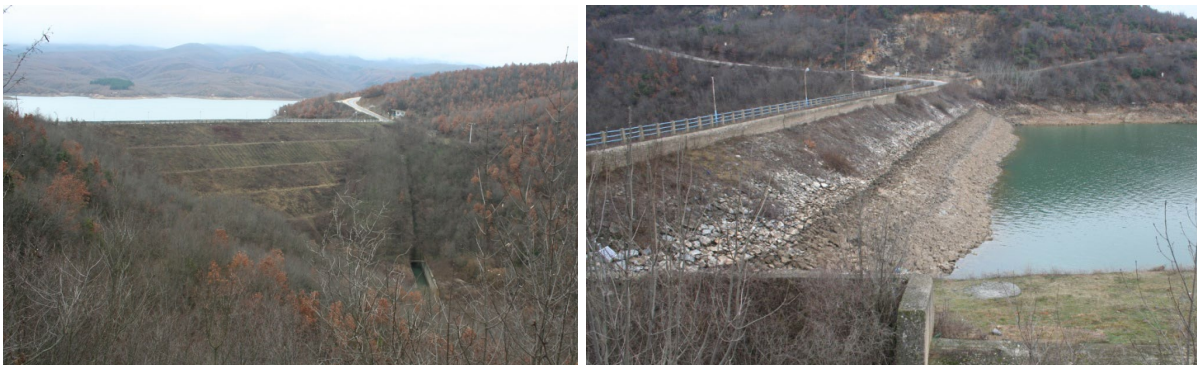
Figure 1: Downstream and upstream slope of the dam.
