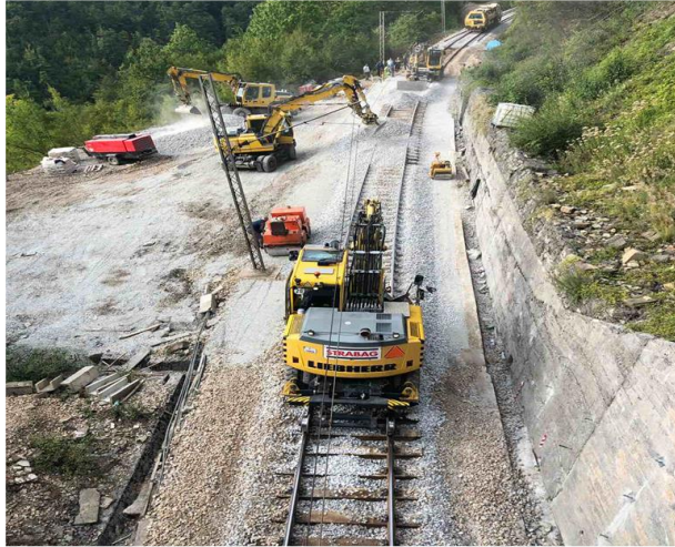
Figure 4. Final works on landslide rehabilitation
