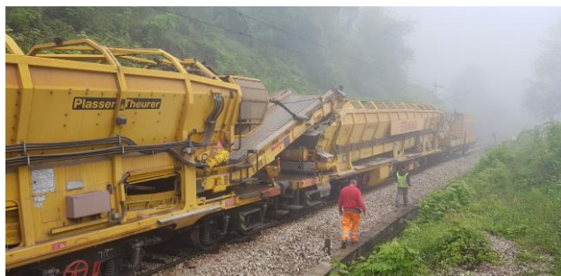
Figure 3 Mechanical ballast cleaning
