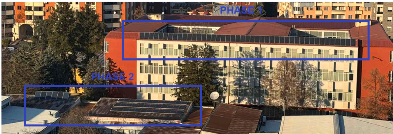
Fig. 2. PVPP at FEEIT, phase 1- 10 kWp installed power, positioned on roof area of building 1 and phase 2, 12 kWp installed power, positioned on roof area of building 2.
