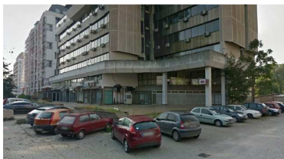
Figure 12. Photograph of the building shown in Figure 10 – north side
