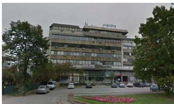
Figure 13. Photograph of the building shown in Figure 10 – south side
