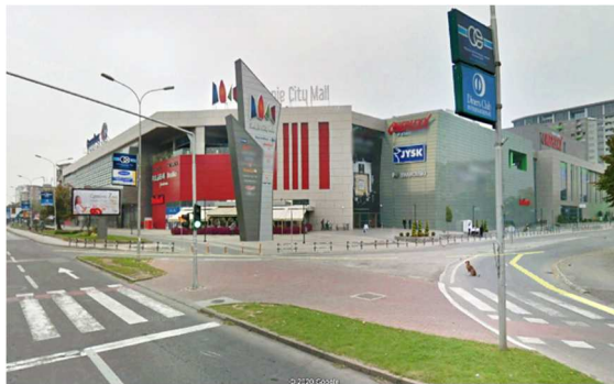
Figure 8. Photograph of the building shown in Figure 7 - Skopje City Mall
