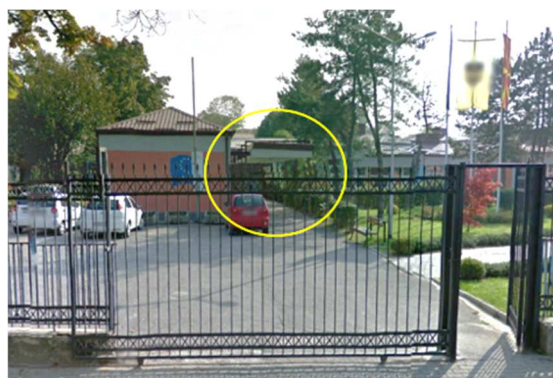
Figure 6. Photograph of the canopy on the building shown in Figure 5
