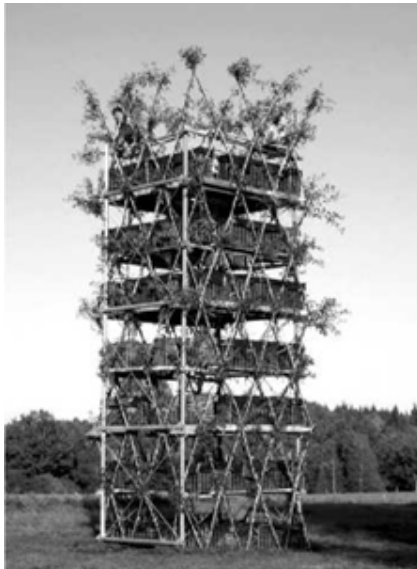
a) Pic. 2 Living tower [7 http://www.dezeen.com/2011/10/25/the-patient-gardener-by-visiondivision/ ]: a) Baubotanik-Turm, b) The principle of building green tower
