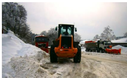
Figure 5. Winter maintenance of mountain saddle Straza (1.150 m altitude) on the national road M-4 (E-75)
