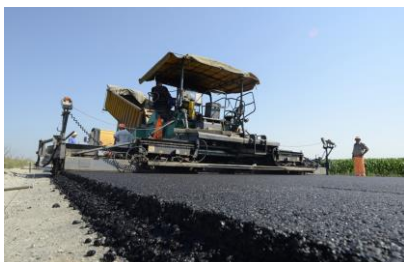
Figure 6. Maintenance of roads (Restoration of surface roads)
