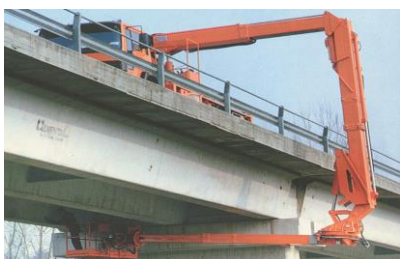
Figure 4. Regular annual reviews of the bridges of the road network
