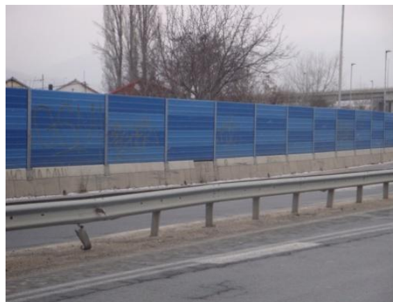
Figure 21. Absorptive acoustic barrier in Skopje
