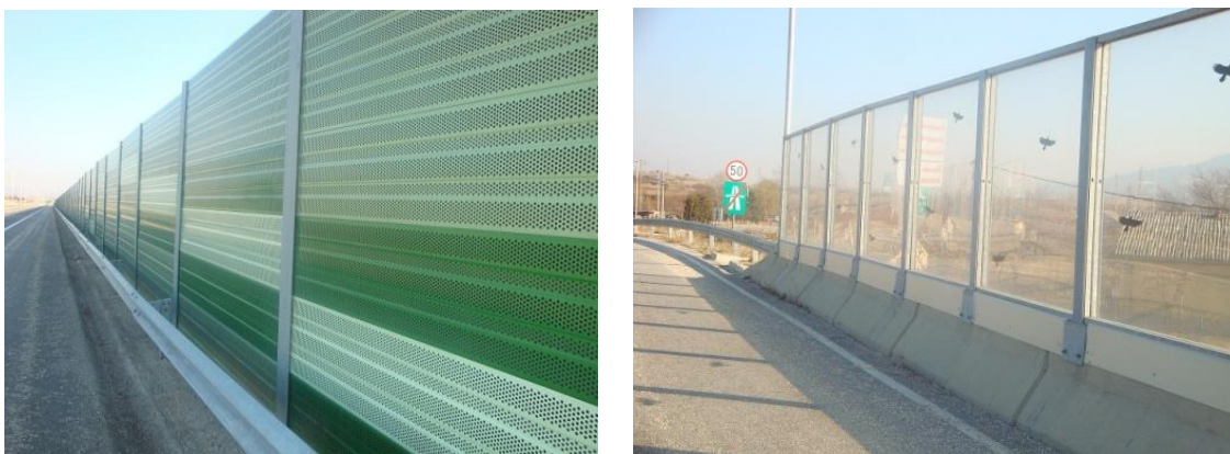
Figure 16 & 17. Absorptive and reflective acoustic barrier at Skopje Ring Road, motorway A-2 (E-75) Source: (own photo)
