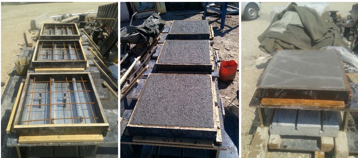
Figure 3. Casting of the concrete for the modified testing specimens
