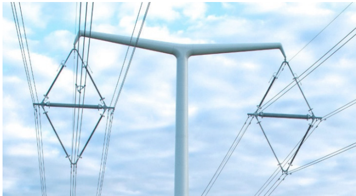
Fig. 2. Steel tubular tower
