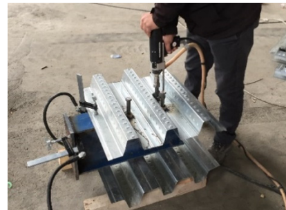
Fig. 2. Welding headed stud through steel sheeting with stud gun
