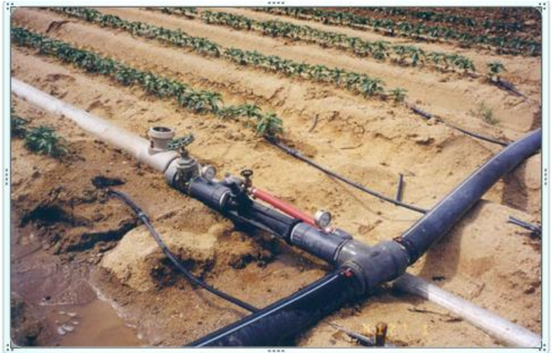
Figure 12 photo of AirJection® system (Mazzei)
