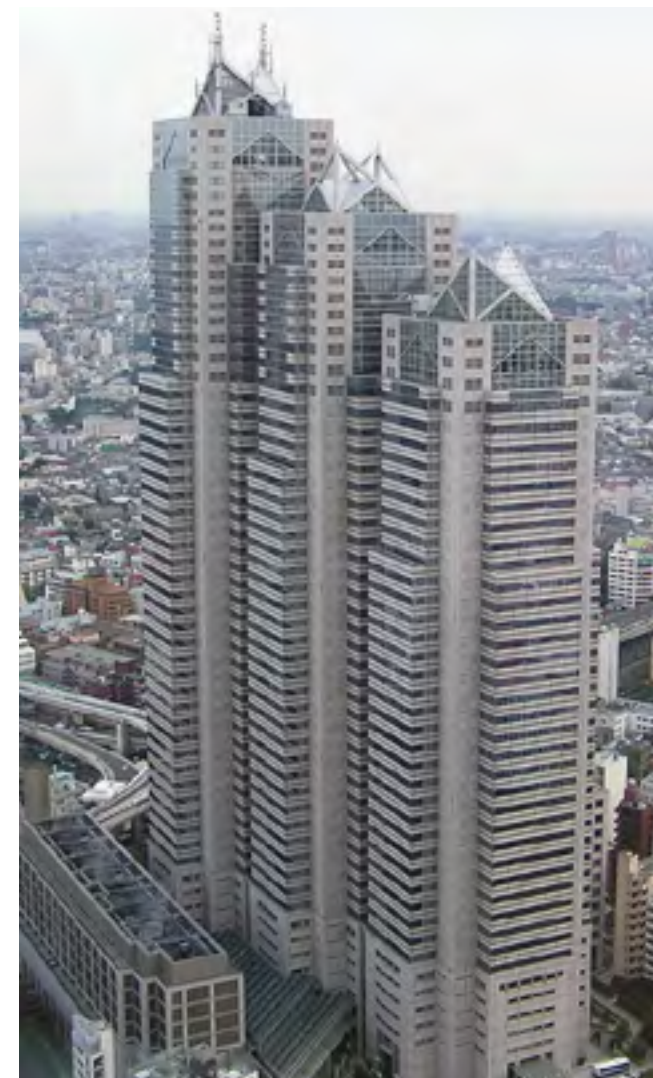
Shinjuku Park Tower. Shinjuku Business District, Tokyo
