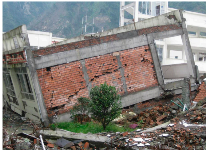
Figure 1. Collapse of a two-story infilled RC building during the 2008 Wenchuan earthquake (photo creator: Zhe Wang) [28].
