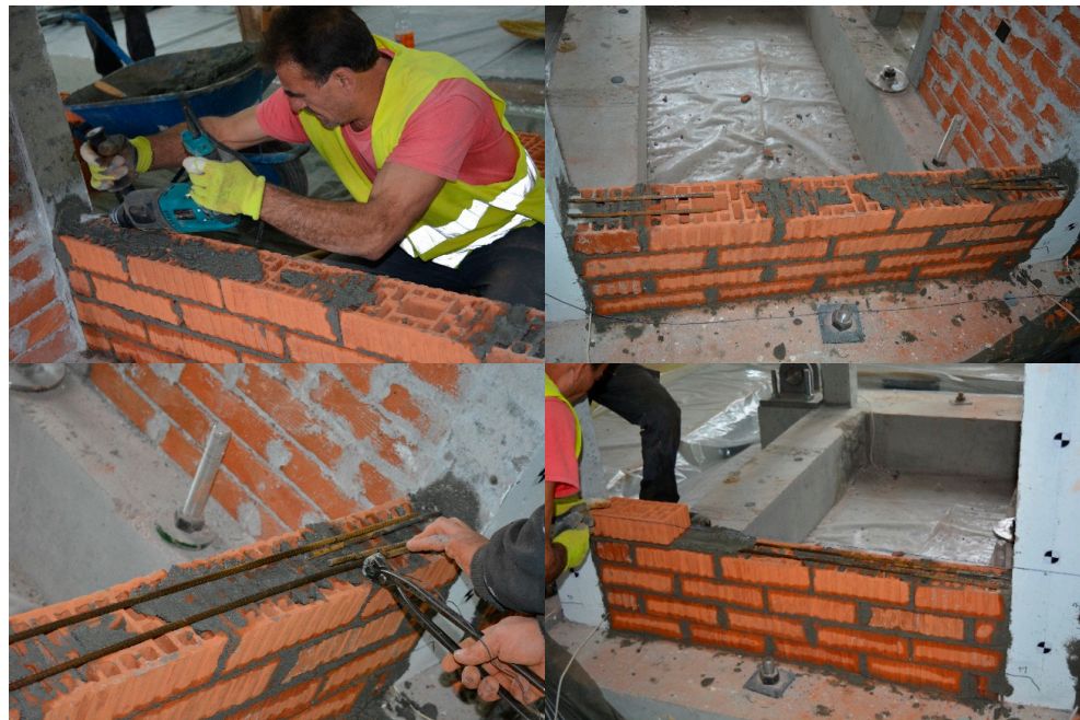
Figure 12. Construction of the proposed connection of Model IW-SB.
