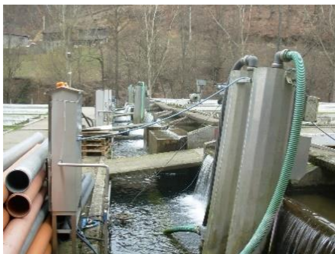
Figure 4. Downflow bubble contactor at a trout farm in Serbia (Photo: S. Čanak, 2007).
