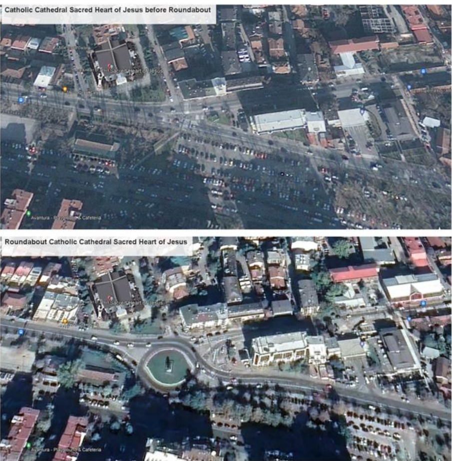
Figure 3. Location of the Roundabout Catholic Cathedral Sacred Heart of Jesus, before and after construction
