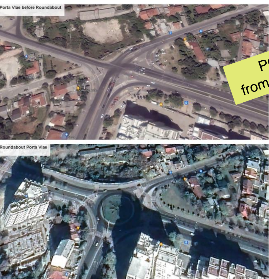
Figure 2. Location of the Roundabout Porta Vlae, before and after construction
