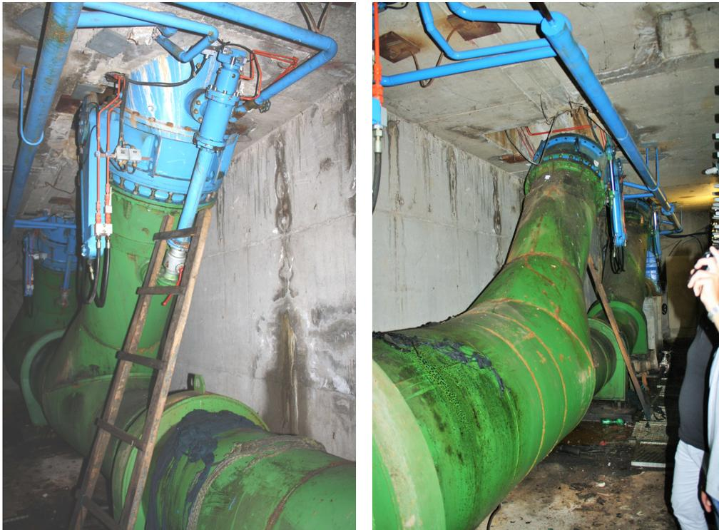
Fig.10. Branches to the turbine unit
