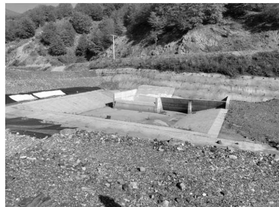
Figure 9. Spillway structure in TSF Sasa 3-2 for evacuation of flood wave from Petrova river
