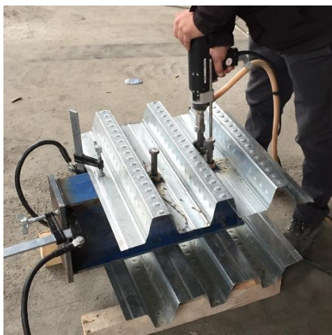
Fig. 2. Shear studs welding process
