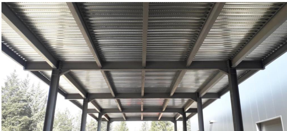
Fig. 1. Constructed composite structure
