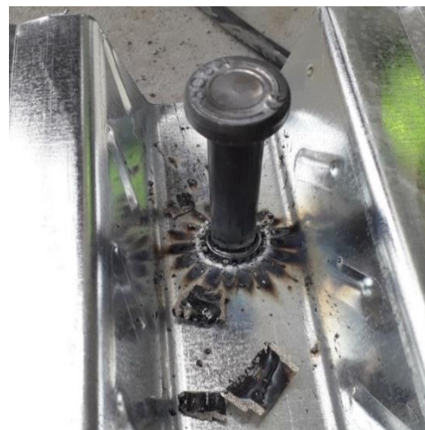
Fig. 3. Through-deck welded stud
