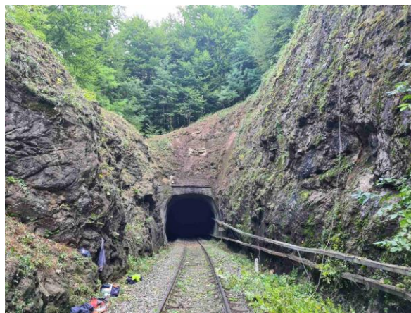
Figure 1. View of the portal slope
