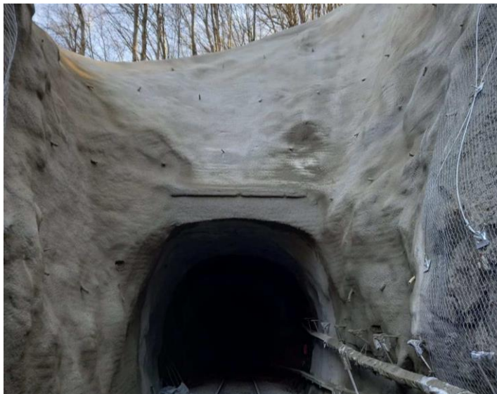
Figure 5. View of the performed portal protection at the Plavce Draga tunnel
