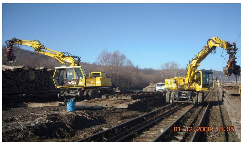
Fig. 2 Special excavators for the dismantling of rail fields
