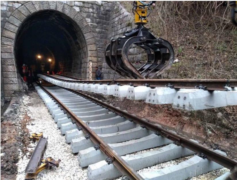
Figure 3. An example of ready-made field's method when it is impossible to utilize a crane due to a lack of space
