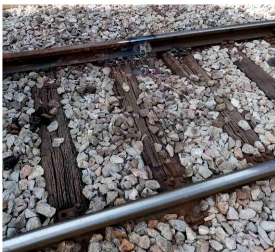
Figure 3. Superstructure with railway track of CWR Source: Prospection in situ
