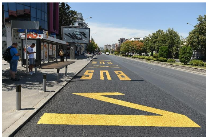
Figure 6. Bus stop on existing carriageway
