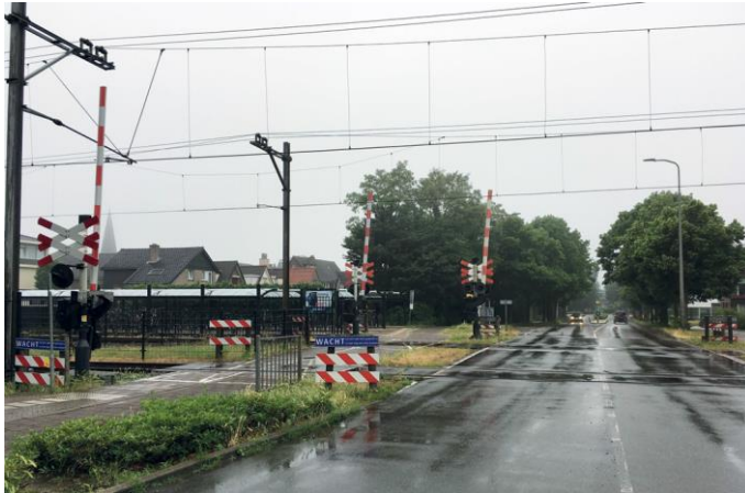
Figure 1. Example of a level crossing in the Netherlands (Dutch Safety Board, Level crossing safety - a hazardous intersection of interests, 2018)
