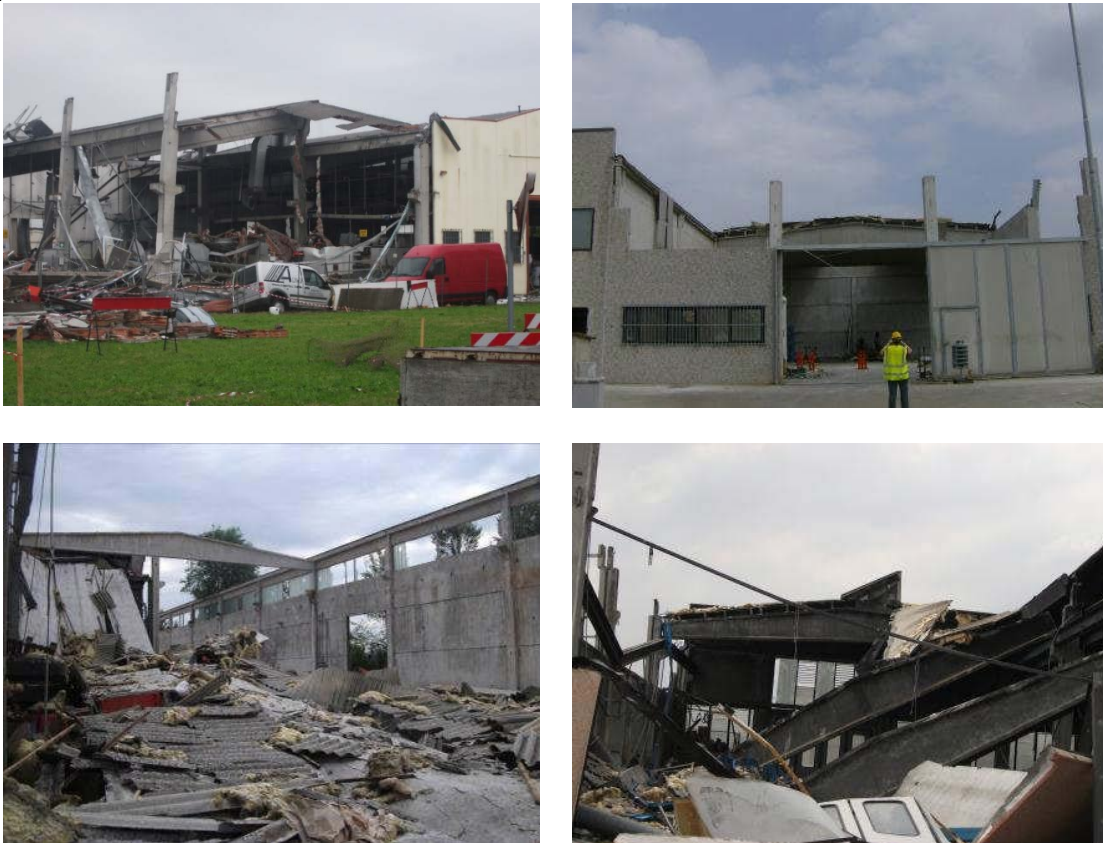
Fig. 2.11 Collapse of beam-to-column connections of precast building due to the Kocaeli earthquake, structural pinned connections.
