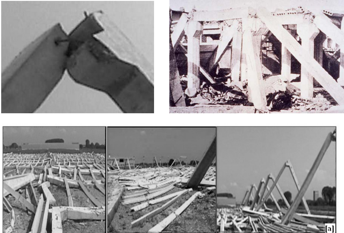
Fig. 2.13 Collapse of a precast building due to various earthquake, mainly due to failure of beam-to-column connections
