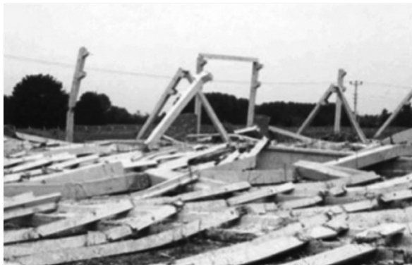
Fig. 2.10 Collapse of a precast building due to the Kocaeli earthquake, where damages at the beam-to-column connections are visible.
