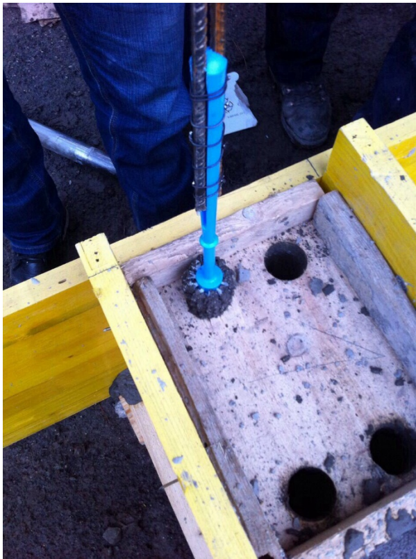
Fig. 4.22 Method used for treating sleeve walls for adequate roughness.
