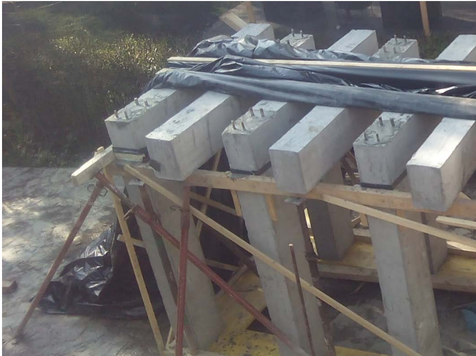
Fig. 4.18. Photo taken during connection of elements with vertically positioned dowels
