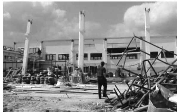
Fig. 2.10 Collapse of a precast building due to the Kocaeli earthquake, where damages at the beam-to-column connections are visible.
