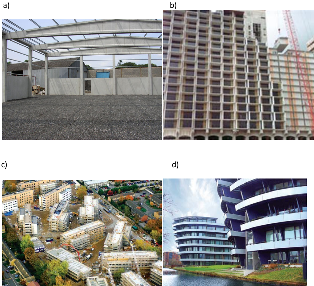
Fig.2.1. Illustration of application of precast structure buildings: a) Typical precast concrete structure building in UK, b) Precast concrete high-rise building in USA, c) Brunel University, Uxbridge, Middlesex – 1400 Students' Room, d) Budenberg building in UK.
