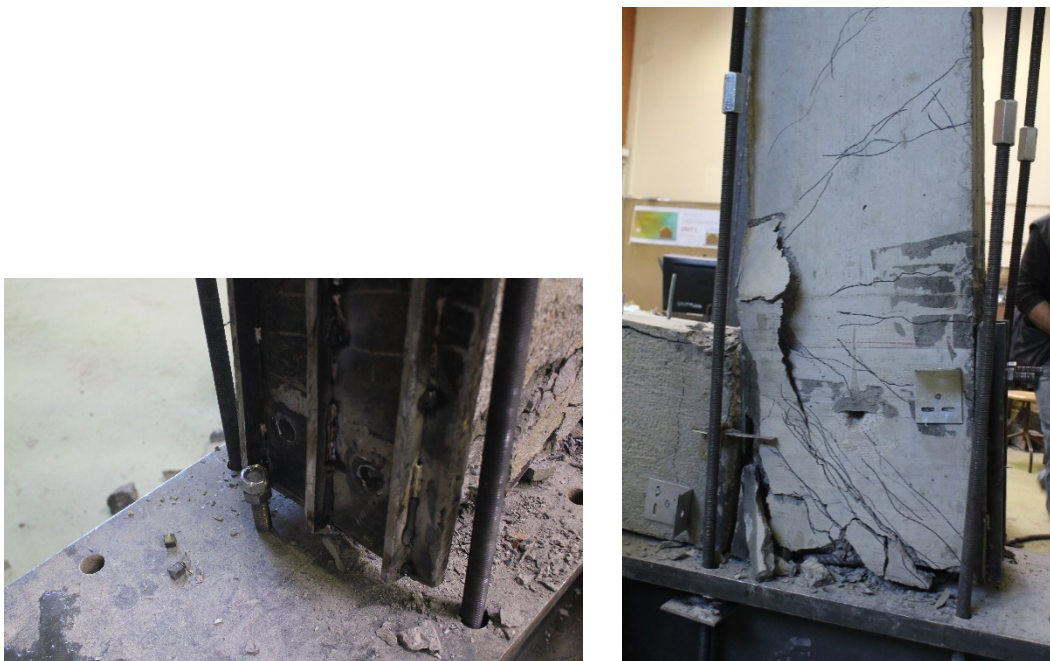
Fig. 4.73 Failure of the joint after the last cycle applied on specimen "S.8 H.D."
