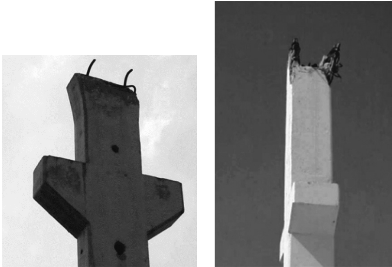
Fig. 2.11 Collapse of beam-to-column connections of precast building due to the Kocaeli earthquake, structural pinned connections.
